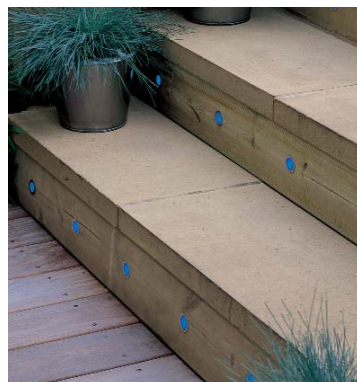
...Illuminate step edges for added safety
